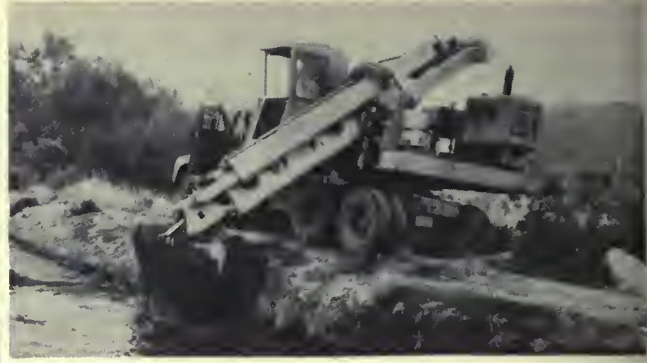
SHAPING NEW DITCH at about 100 feet per hour, left. Above, removing moss and silt at rate of 1 mile per day per machine. All photos by the author.
